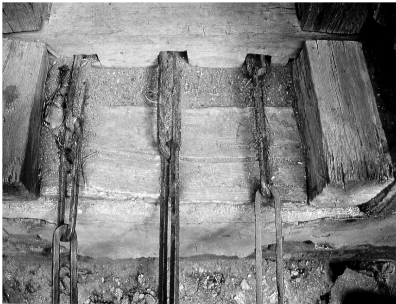
Fig. 35: The anchorage of the Doksum Chakzam
