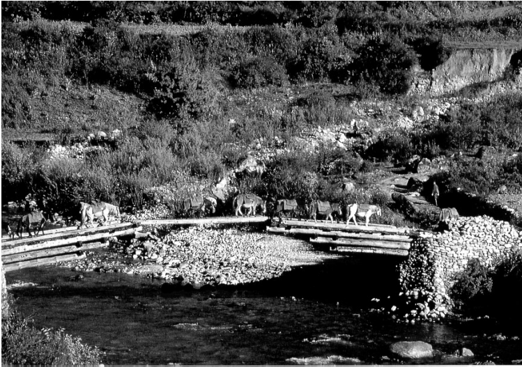
Fig. 24: Horse caravan on the former cantilever bridge across the Paro Chhu below Taktshang.
