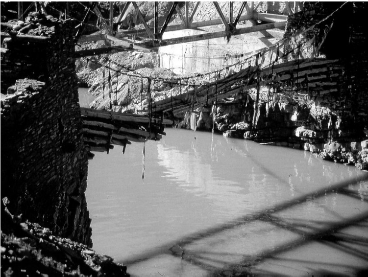
Fig. 28: The combined cantilever and iron chain bridge on the way to Tholing.
