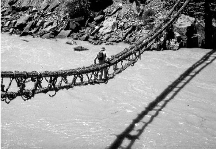
Fig. 22: The author in 1975, on a bridge made from willow tree branches in Ladakh.
